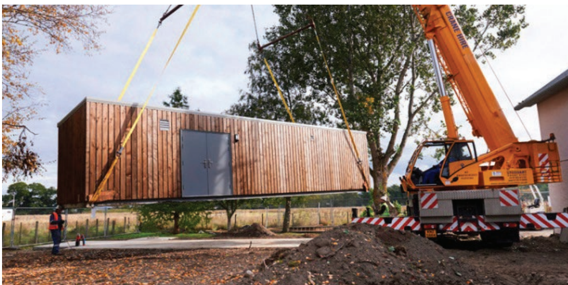
FIGURE 5 Installation of a containerized system
