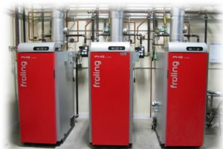
Pellet Boilers/ U.S. Forest Service WERC
